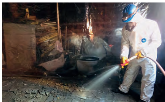
REMOVING TILES CONTAINING ASBESTOS DURING THE RECYCLING OF M/V SALARUM
