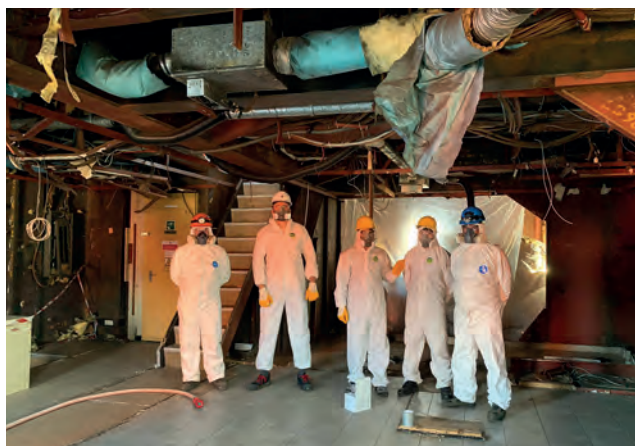
ASBESTOS REMOVAL TEAM WITH APPROPRIATE PPE
